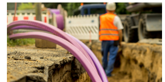
12 to 14 bar: Cable blowing and drilling
