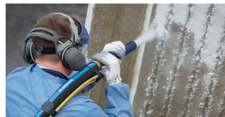
8.6 to 10 bar: Abrasive blasting
